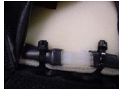
Replacement tie wrap in place.
